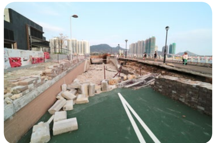
圖三：將軍澳海濱單車徑被風暴潮和巨浪沖毀(岑智明攝) Figure 3: Cycling trails at Tseung Kwan O waterfront was destroyed by storm surge and high waves. (courtesy of Shun Chi-ming)
